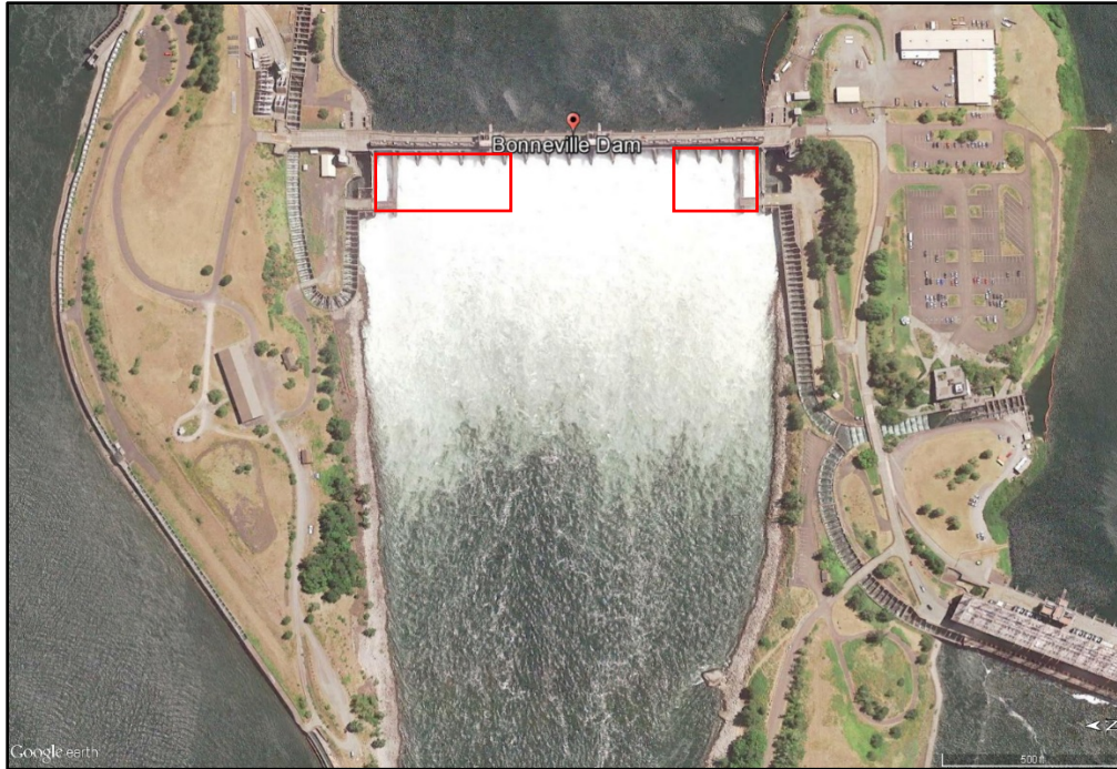
Figure 2 BON Spillway. Red boxes indicate approximate area of inspection coverage.
