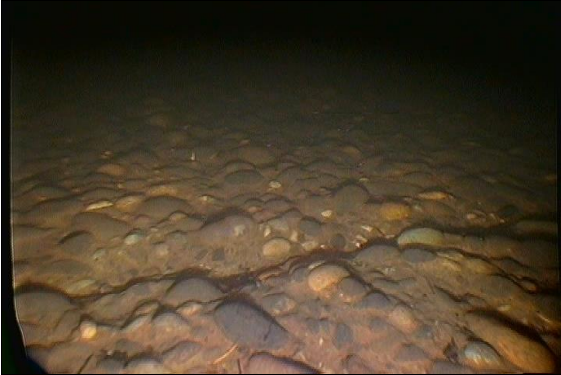
Figure 14 Bay 18 construction joint and apron erosion.
